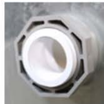
Outside pool wall with lock nut.
