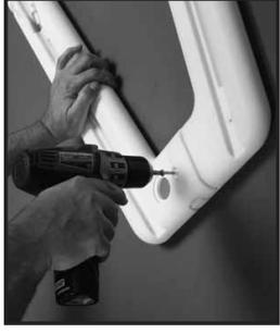
**#2:** Connect the top of the rails together using two #10 x 1-1/4" self-tapping screws (one in the designated mark on the inside rail and one on the outside rail).
