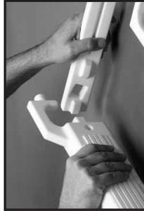
**#2:** Starting at the bottom, rotate one tread connector on edge. Align the square tab on the locking slide tread with the square hole in tread connector.
