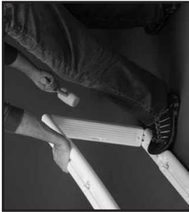
**#8:** Align the remaining notch in the bottom of the rail assembly with the tab of the bottom tread and tap in until firmly seated.
