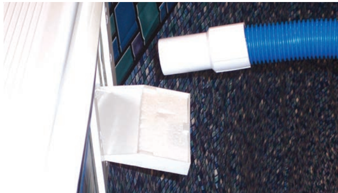
Figure 3 - Positioning weir for vacuuming
